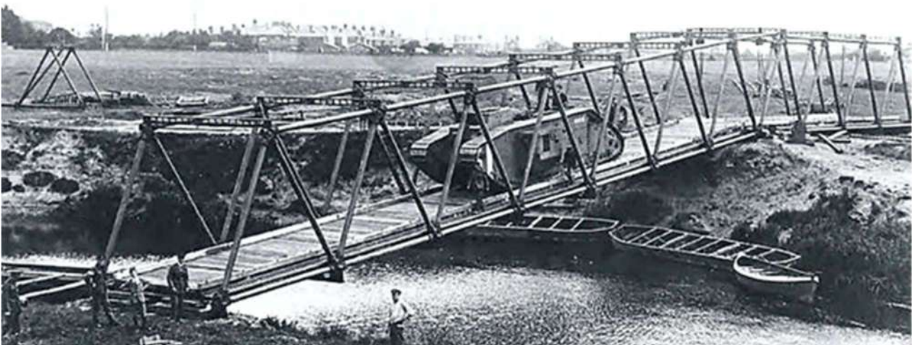
FIG. 9 - ERECTING A TANK BRIDGE WITH A DERRICK
